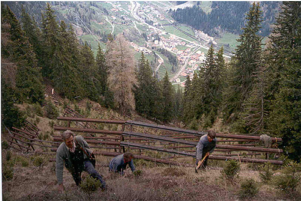
Figure 2. High-elevation afforestation in an avalanche starting zone, controlled by snow-pack stabilizing structures. Forest can take over the functions of the technical measures in the long run.
